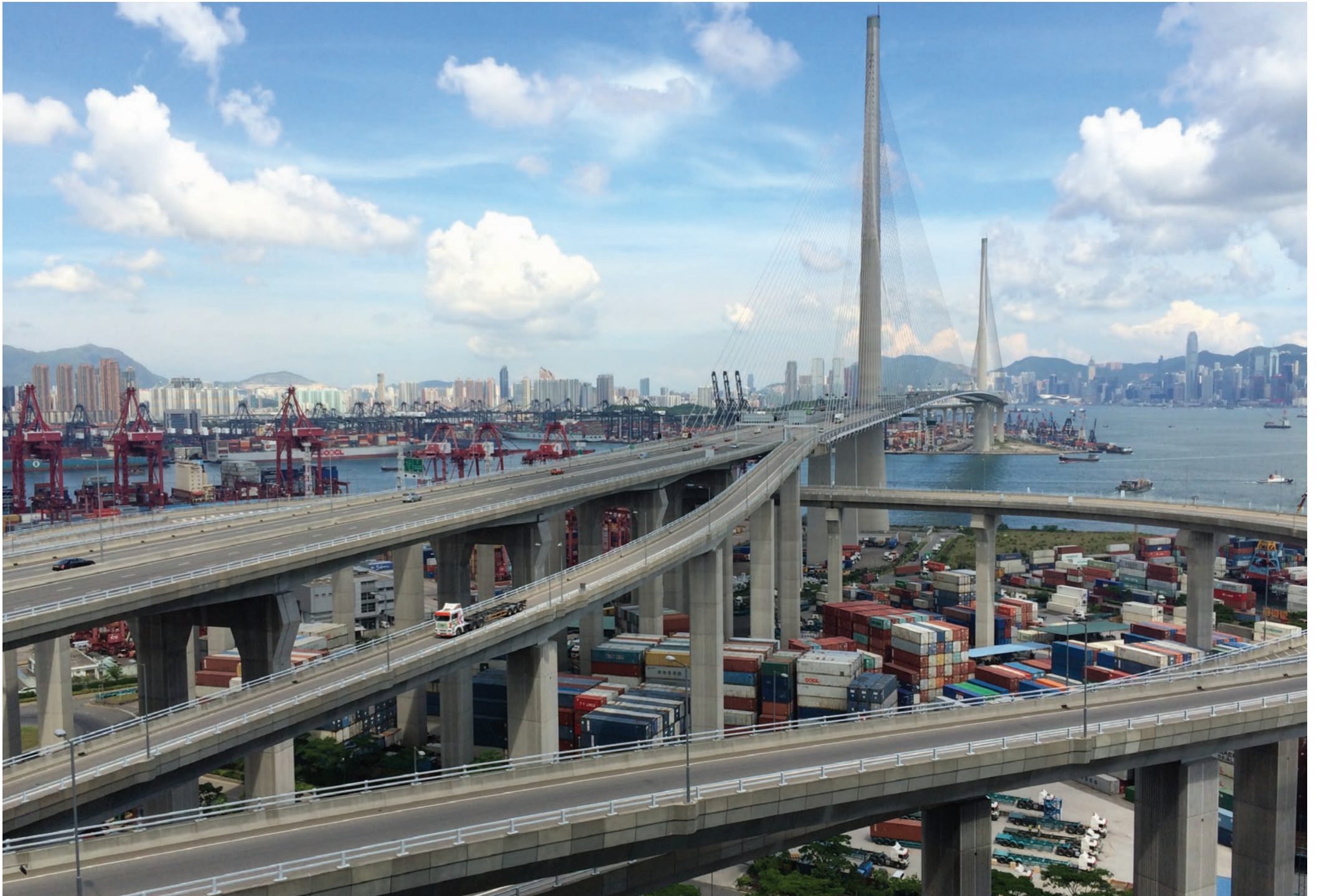
Roof top view from Interlink Mega Hub – Container Terminal 9.
